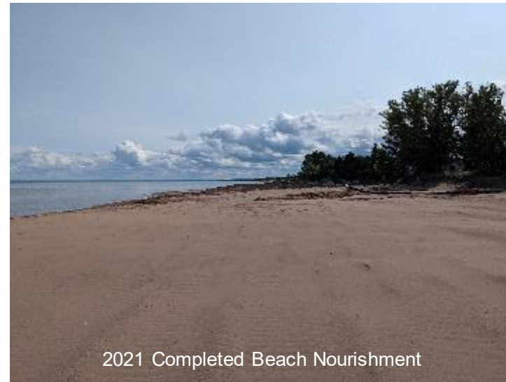
2021 Completed Beach Nourishment
